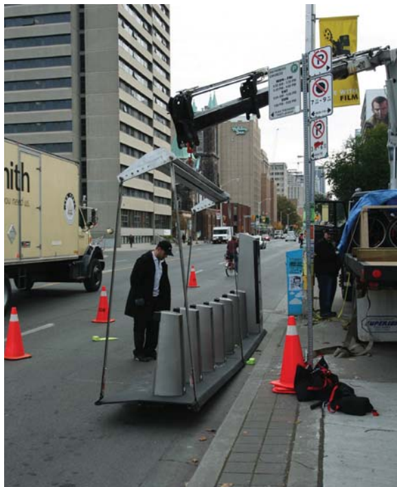
Bixi stations are lifted into place with a boom truck and are bolted to the ground. No excavation is required. Image: Yvonne Bambrick/ysuchislife ( www.flickr.com )
