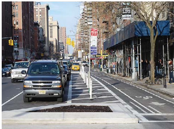
NYCDOT's protected on street bike lane on 9th Avenue in Manhattan. Image: NYCDOT
