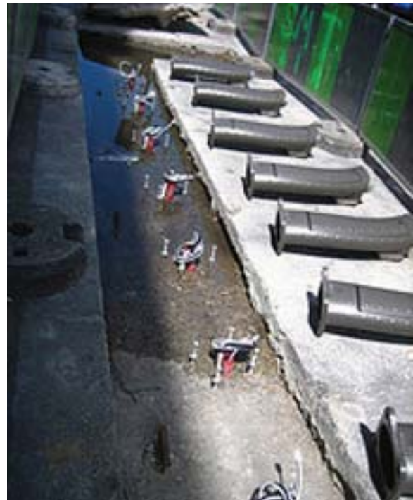
Excavation and trenching is required for JCDecaux (above) and ClearChannel Adshel bike-share kiosks. Image: Ladybadtiming ( www.flickr.com )
